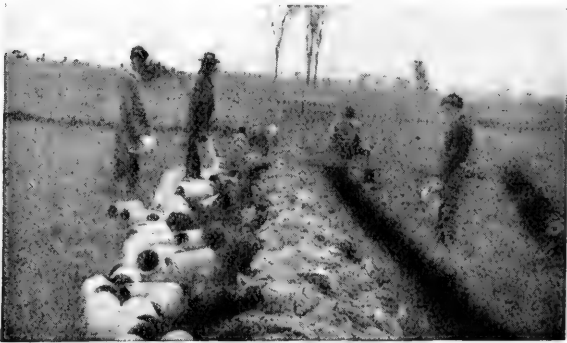
FIG. 38.—Ready to lay the six-inch drain tiles.
